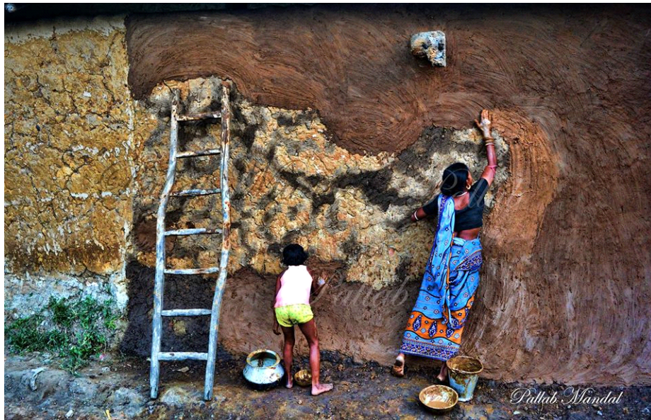
Figure 1: Renovation of the mud wall (Mandal, 2016, October 25).
